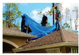
Roofing contractors install FEMA supplied blue tarp sheets onto a Naples, Florida home in order to provide a temporary solution for residence housing shelter and prevent further damage after Hurricane Irma.
