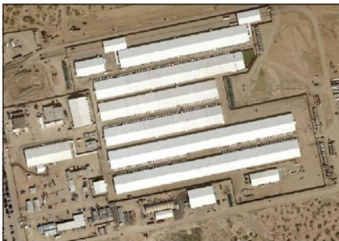
Aerial photo of Camp East Montana
