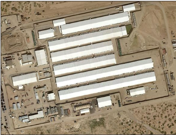
Aerial photo of Camp East Montana
